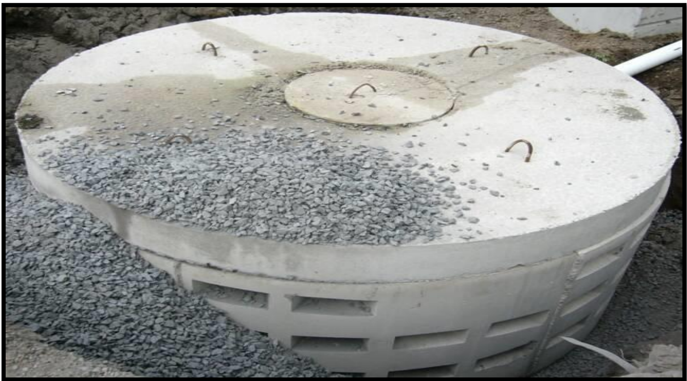
Figure 28. Stormwater Infiltration Well
