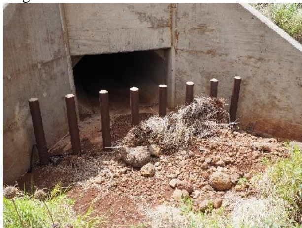
Sediment and Gravel at Culvert Entrance
