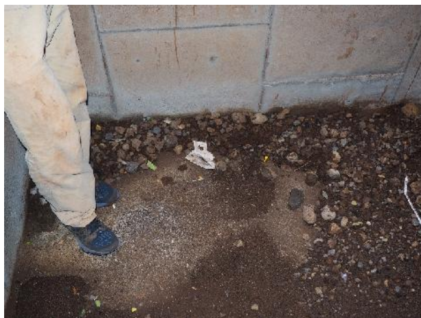
Sediment and Gravel in Culverts
