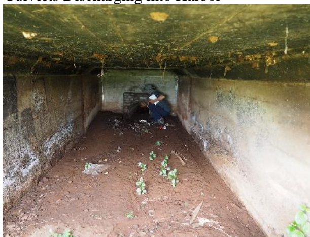
Substantial Sediment Deposition in Culvert
