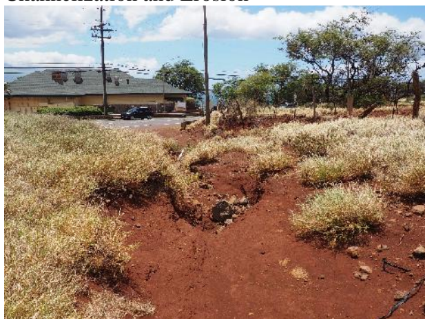
Failed Road with Channelization and Erosion
