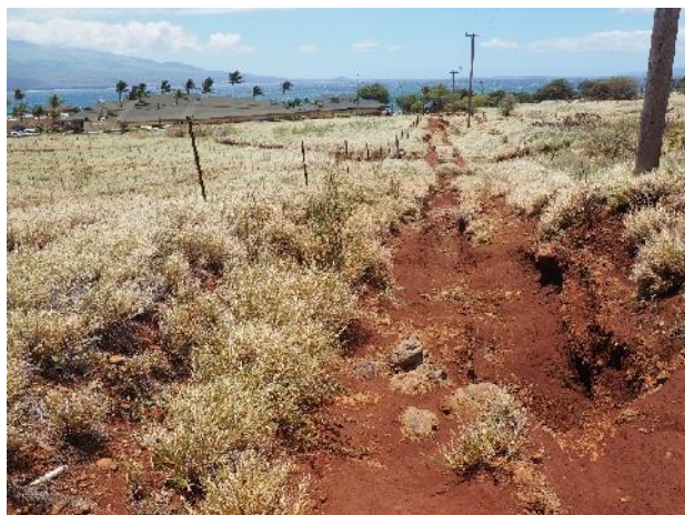
Failed Road with Channelization and Erosion
