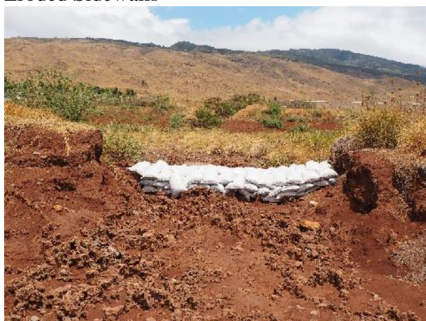
Failed Control Structure
