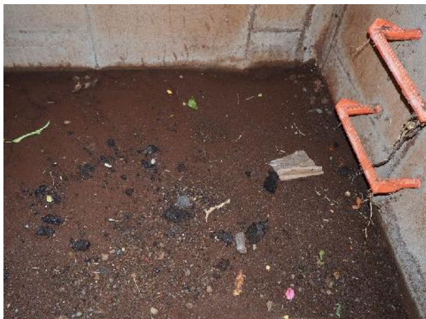
Sediment and Gravel in Culverts
