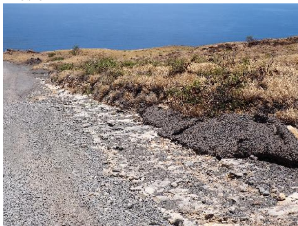
Gravel Loss in Swale
