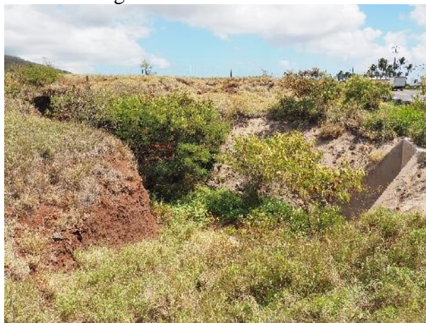
Culvert Backwall and Head Cutting
