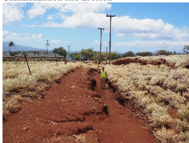
Failed Road with Channelization and Erosion
