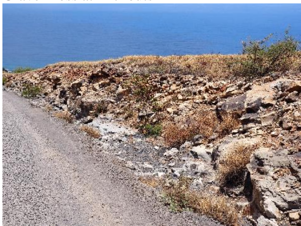
Channelization and Gravel Loss in Swale
