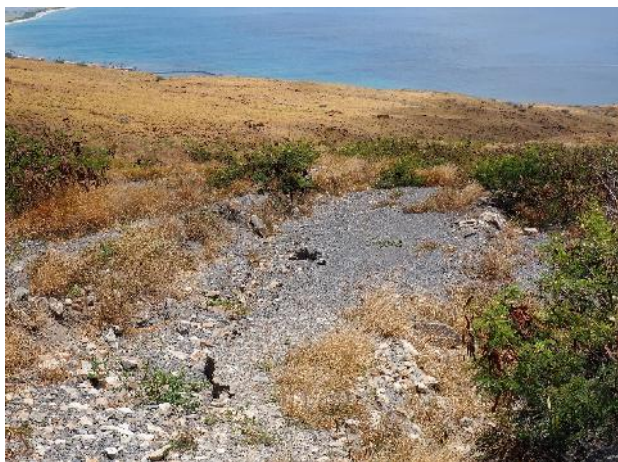
Gravel Loss at Kickouts
