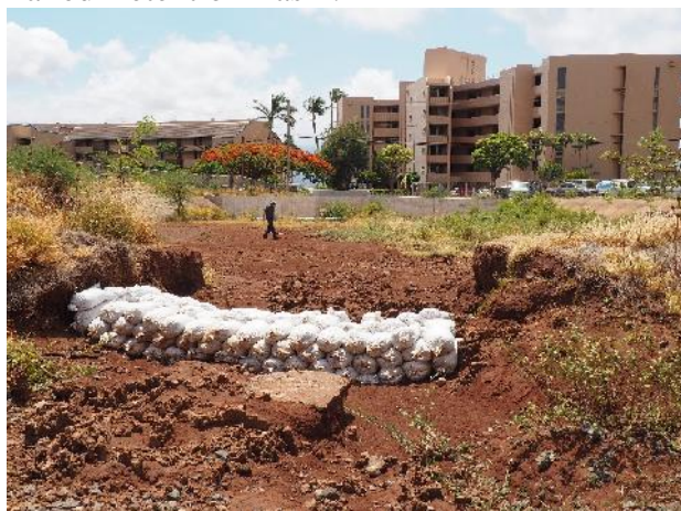
Sand Bags at Failed Control Structure
