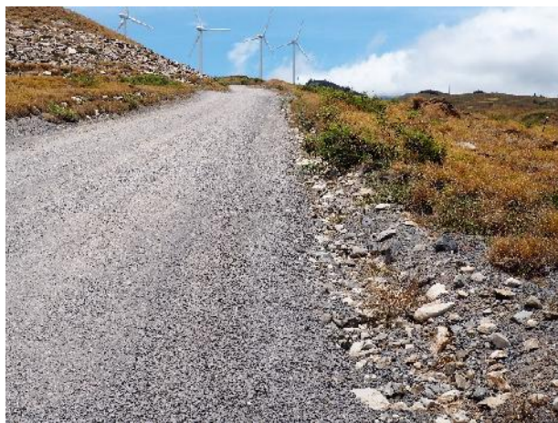
Well Maintained Road with Swale
