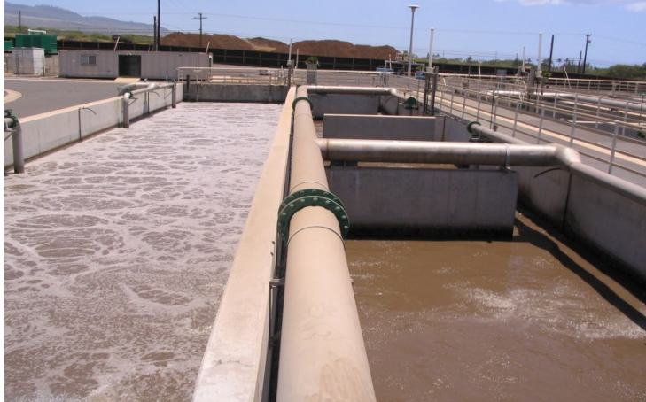
Figure 3: Kihei WWRF Flexible Aeration Basin
